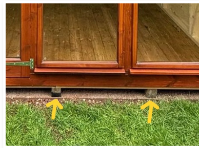
3"x3" tanalised timber bearers for air circulation under building
