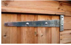
Security (frame bolted)
