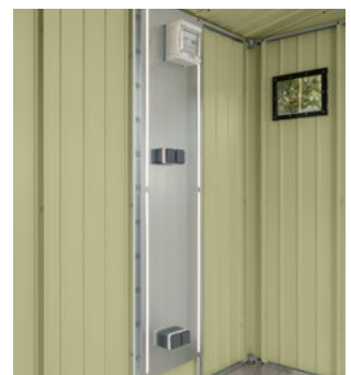
Electric panel incl. sockets and LED lighting, without optional power connection Width x height: 47 x 180 cm
